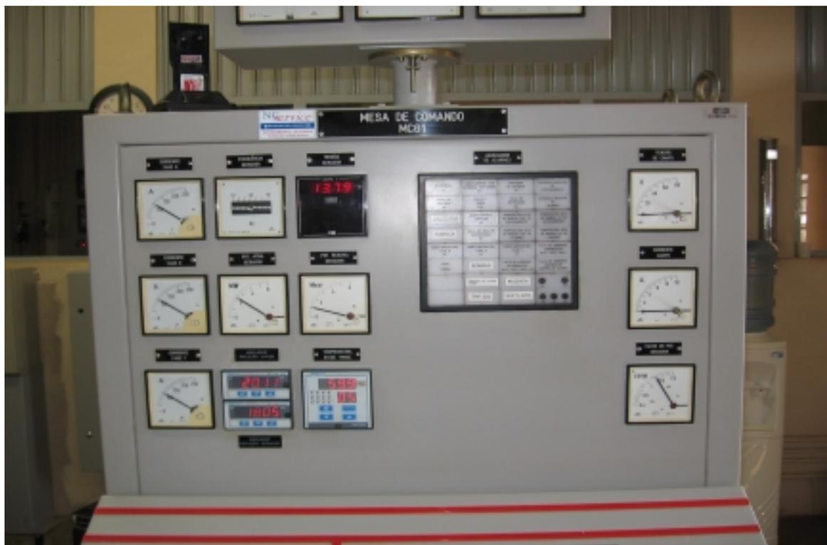
**FOTO 8 – EQUIPAMENTO REGULADOR DE TENSÃO NA SALA DE COMANDO DA GERAÇÃO ELÉTRICA**
